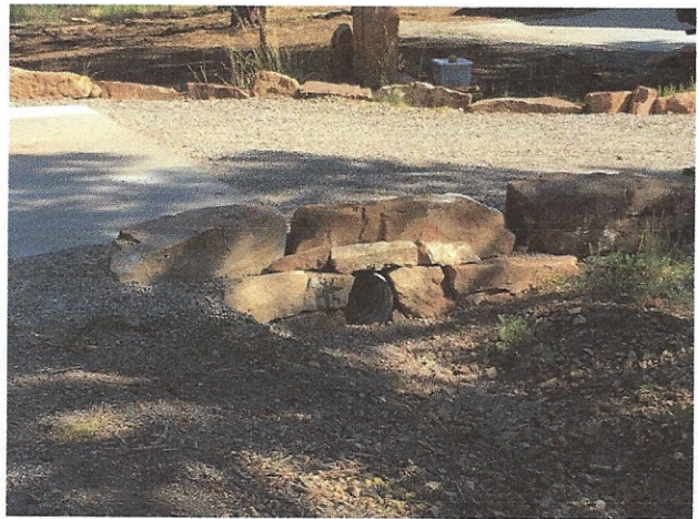
Lot V612 culvert end - South side
