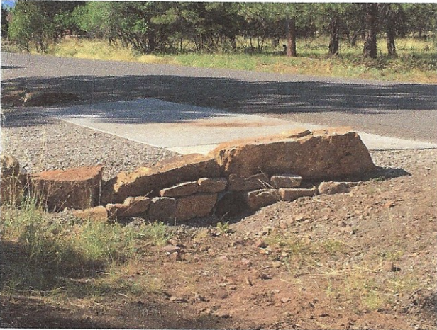
Lot V612 culvert end - North side
