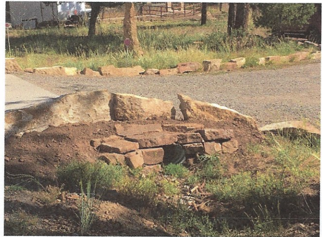
Lot V613 culvert end - South side
