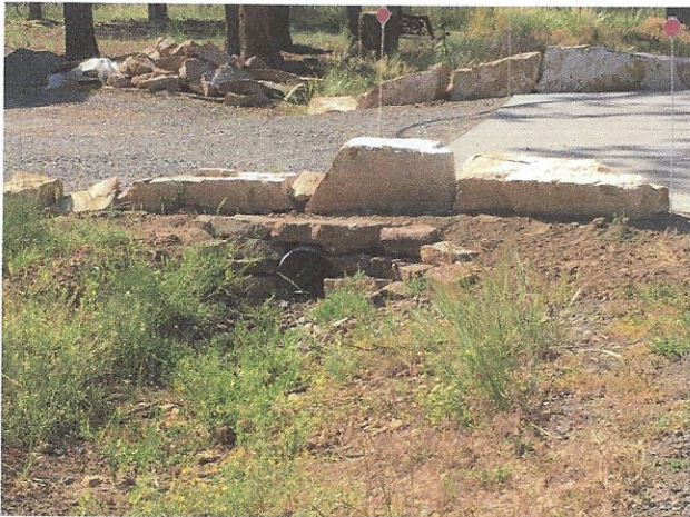
Lot V613 culvert end - North side
